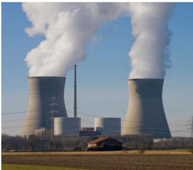
The Gundremmingen plant is run by the German utility RWE
